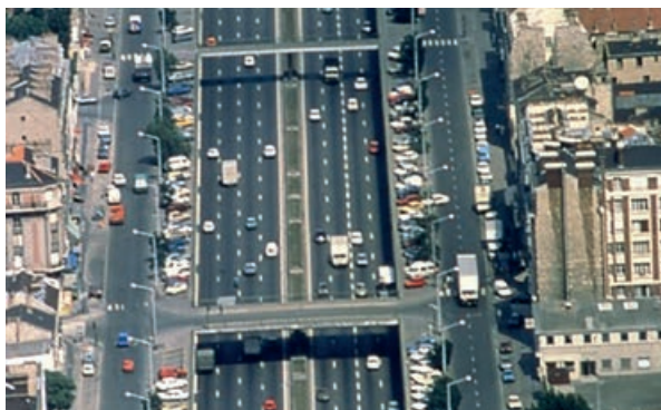
Photo 3 - Autoroute A1 avant requalification.
