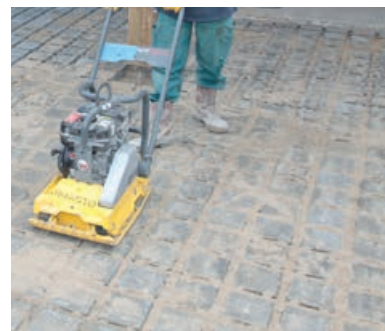
Photo 83 - Damage des joints.
